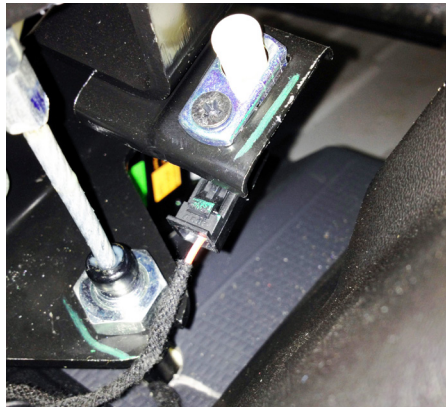
Figure 4. View of Park Brake terminals
